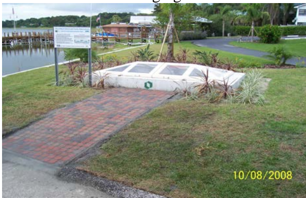
Nutrient Separating Baffle Box with Glass Top & Sign
