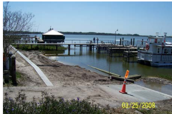
Lakefront After Dredging & Seawall
