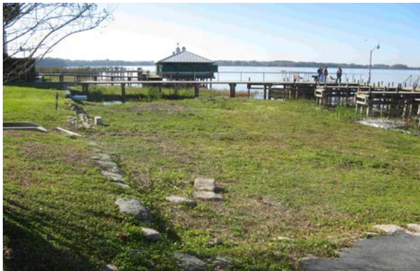
Lakefront Before Dredging & Seawall
