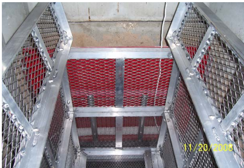
NSBB Installed Inside Existing Box Under Sidewalk
