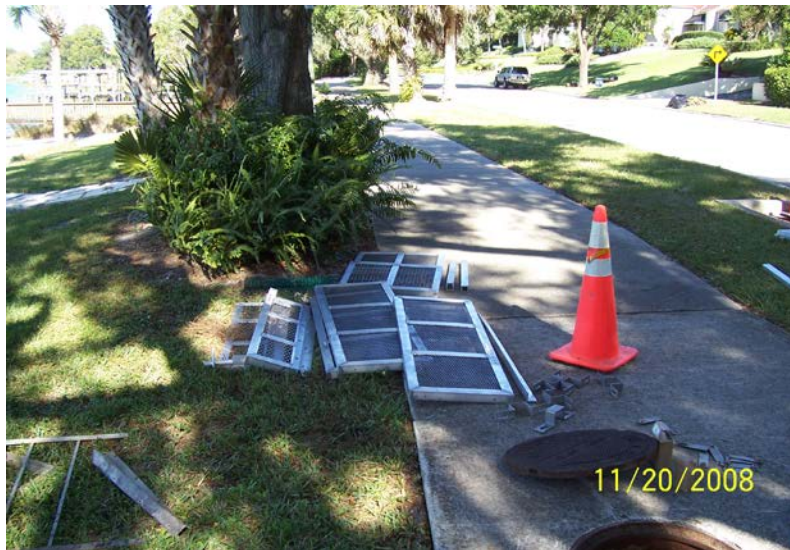
Parts of the NSBB Installed Under Sidewalk at Lake Gertrude
