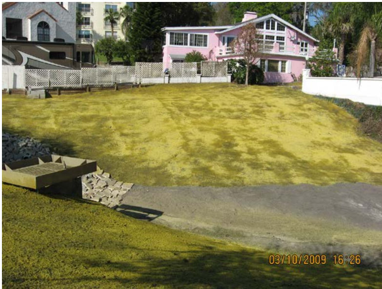
Retention Pond at Old 441 Repaired and Hydroseeded
