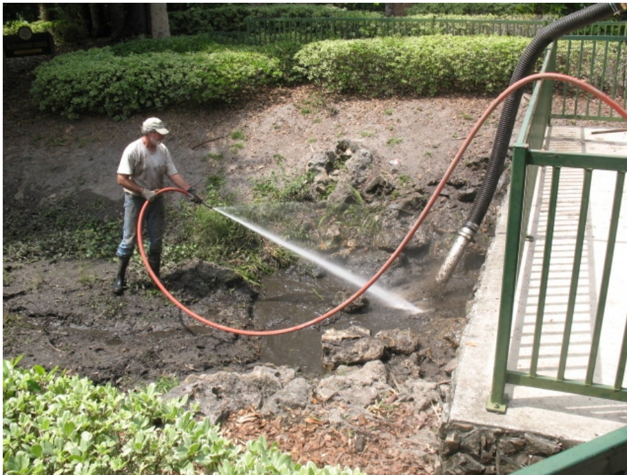
Jet and Dredging of Alexander Creek Upper Pond
