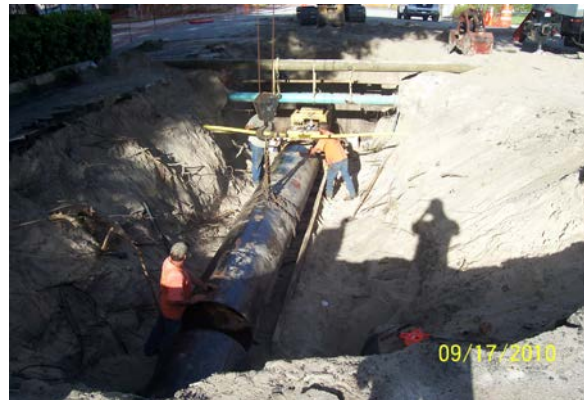
Steel casing with auger being set in place
