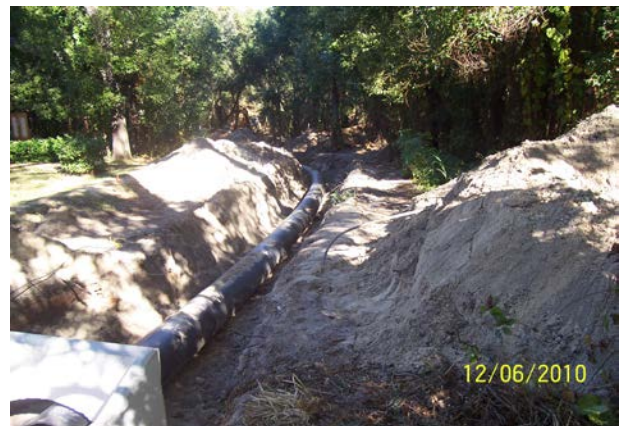
Stormwater pipe installation
