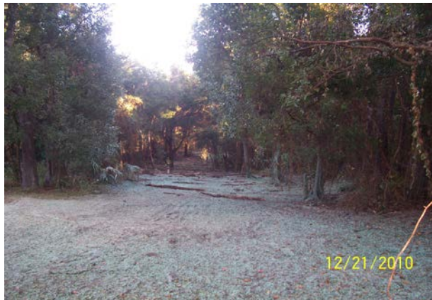
Hillside restored and hydroseeded
