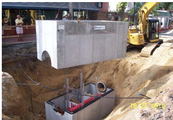
Top section of baffle box being set in place
