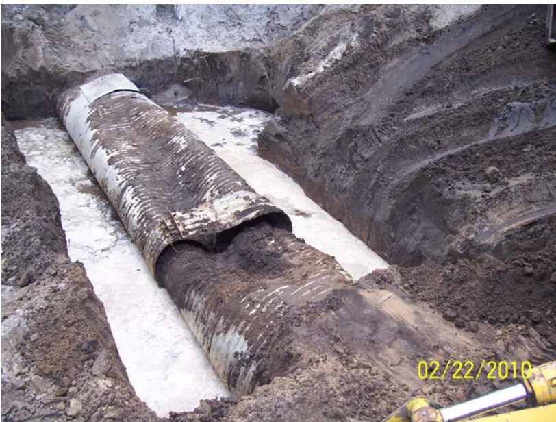
Excavation of crushed section of pipe
