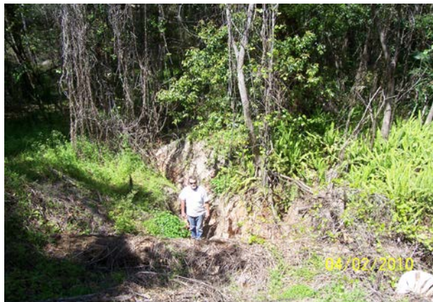
Erosion down hillside before construction
