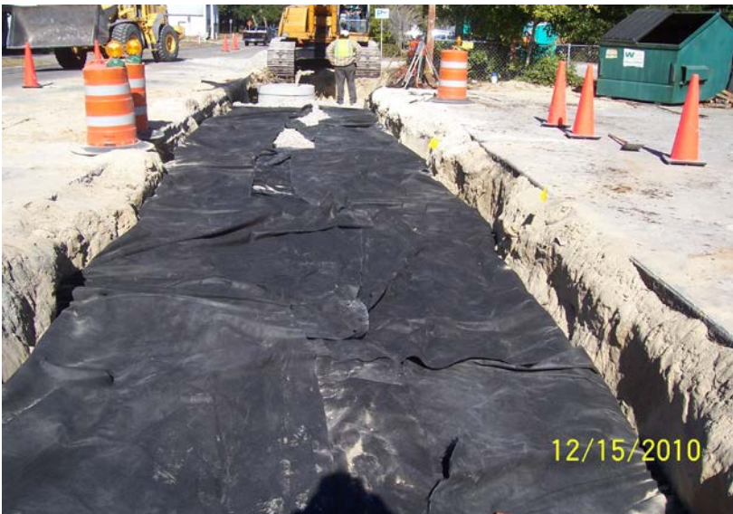
Chambers surrounded with stone and filter fabric
