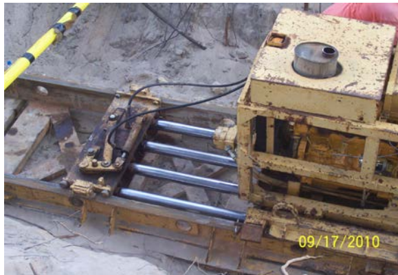
Hydraulic rams for Jack & Bore
