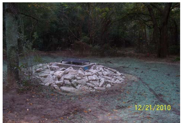
Discharge structure at base of hill
